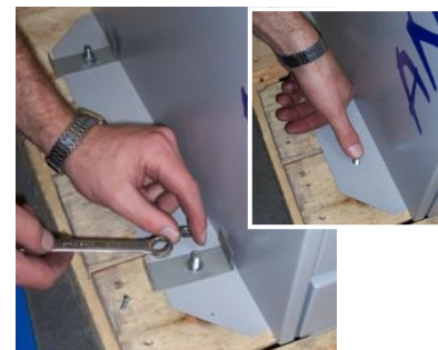
2. Release & Remove the transit bolts (see insert).
